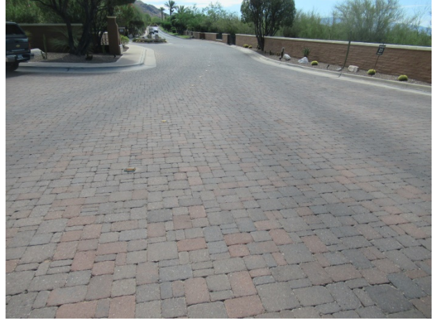
Vehicular pavers near gate house
