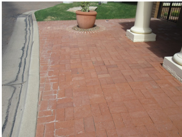
Pedestrian pavers in front of office building
