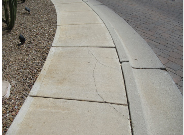
Sidewalk cracks
