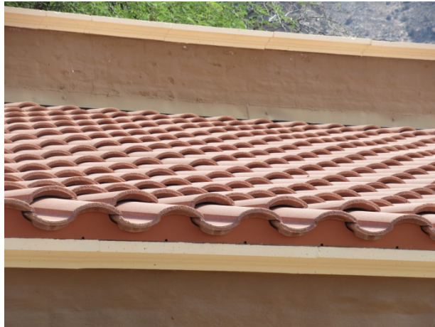
Concrete tile roof
