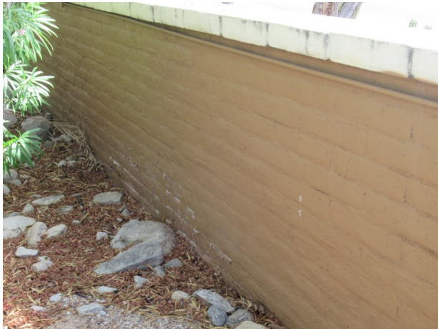
Paint deterioration
