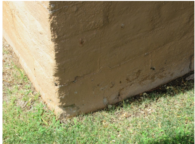
Masonry deterioration
