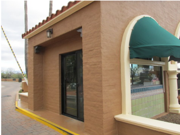
Gate house stucco and paint finish application overview
