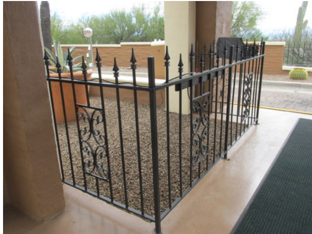
Metal fence at gate house
