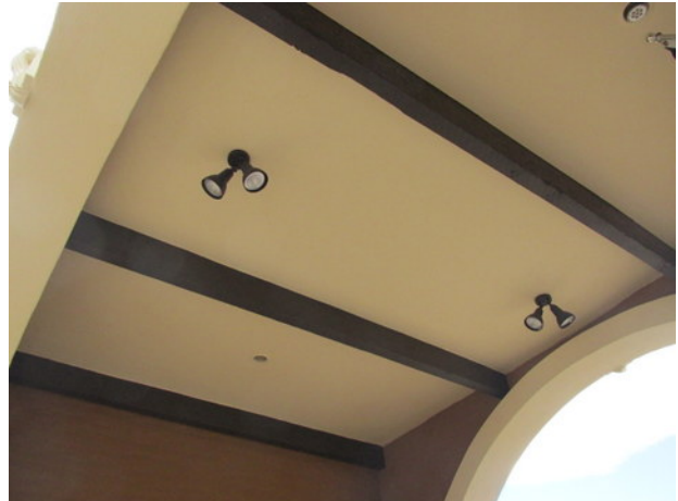
Gate house overhang underside
