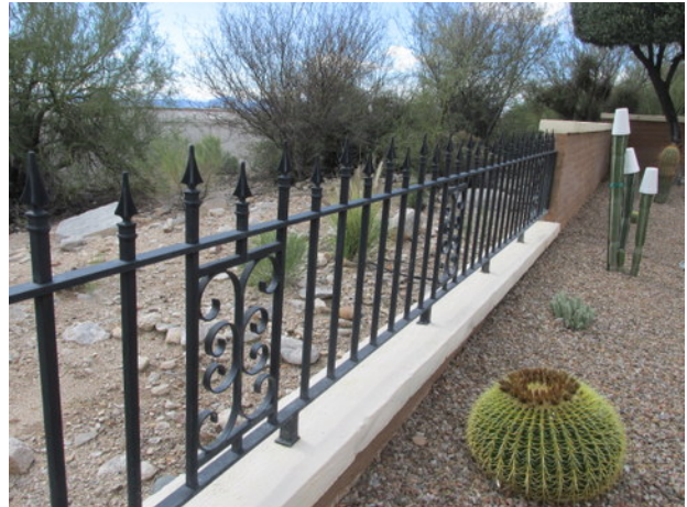
Metal fence along perimeter wall
