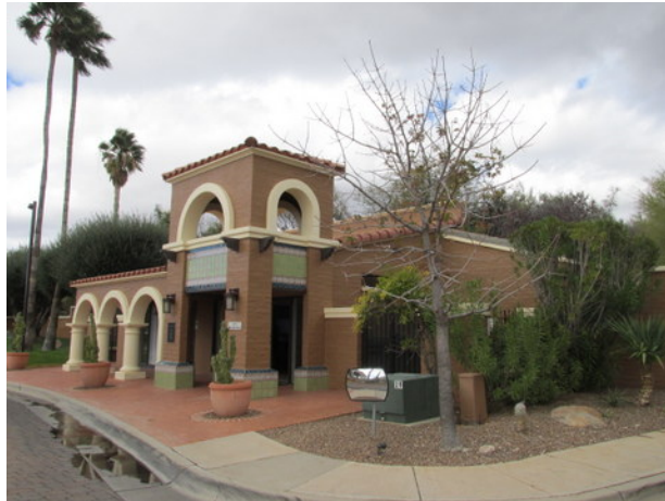
Office building stucco and paint finish application overview
