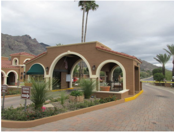
Gate house front
