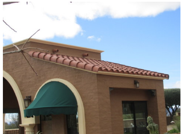
Gate house concrete tile and flat roofs
