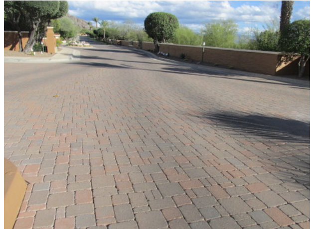
Masonry pavers along Ina Road
