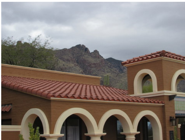
Office building concrete tile roof
