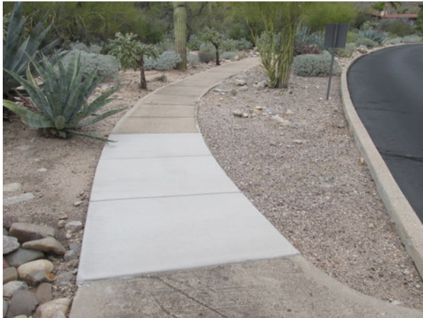
Concrete sidewalk partial replacements near office building and gate house area
