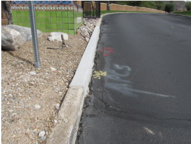
Concrete curb replacement near community entrance
