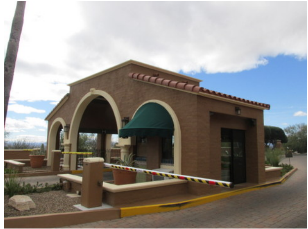
Gate house rear
